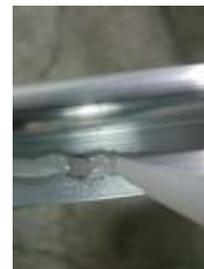
4. To attach the side aluminium profiles, remove the red backing tape from the underside of the profile. Locate the Side Extrusion (1350mm) hard up against the front edge of the tub with the notch to the rear. Slide each the profile down keeping the taped surface square with the top of the tub. Press down firmly to ensure adhesion.
