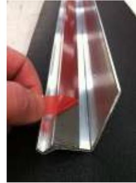
5. Using the PVC drill templates locate the templates along the bottom edge of alloy, mark the locations onto alloy. With a 4mm drill bit, drill each of the locations through the aluminium and into the inside edge of the tub.
