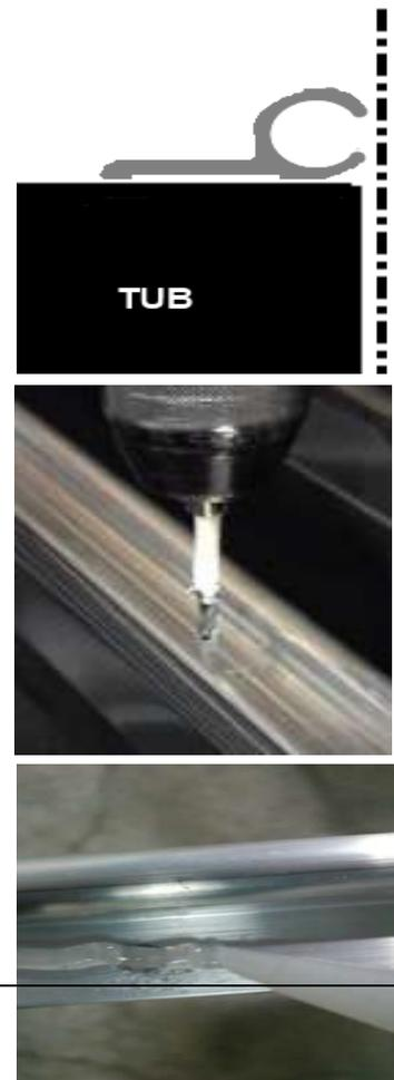
9. To attach the side aluminium profiles, remove the red backing tape from the underside of the profile.
